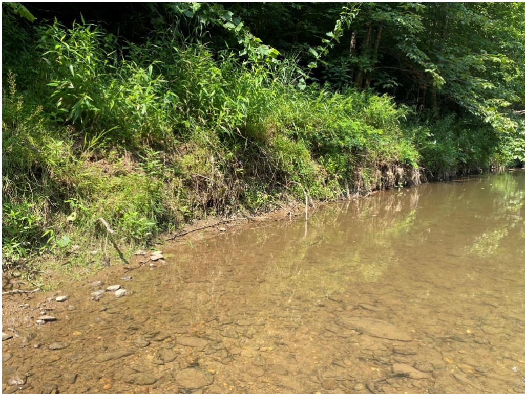
Erosion Area 10; Category “Moderate”
