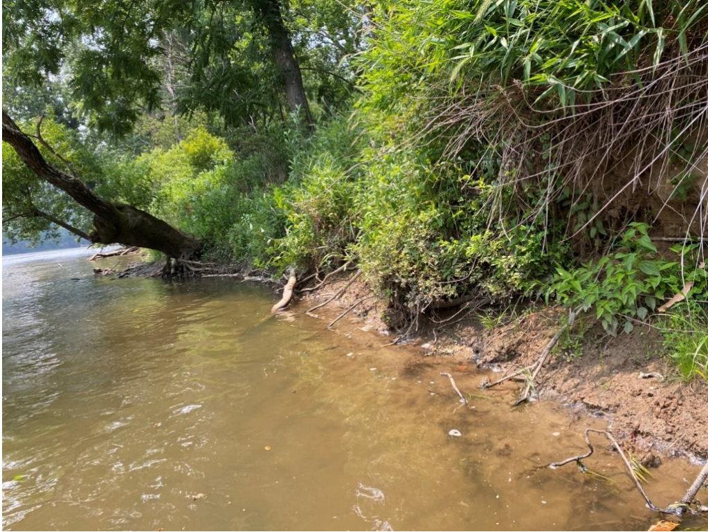
Erosion Area 5; Category “High”
