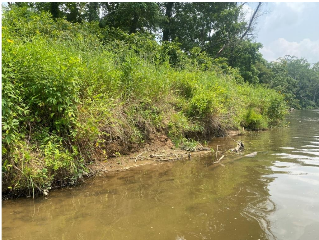
Erosion Area 4; Category “High”
