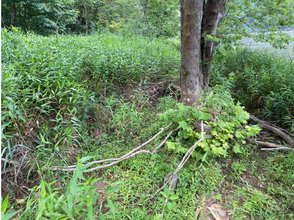
Erosion Area 15; Category “Low”
