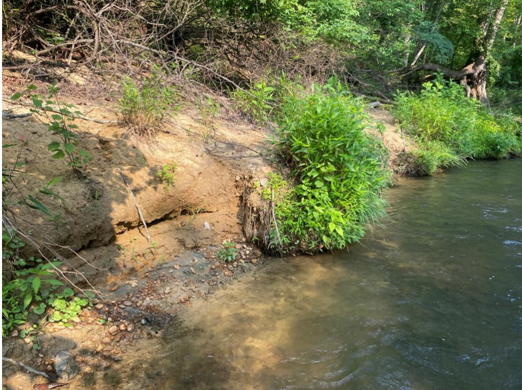
Erosion Area 1; Category “High”
