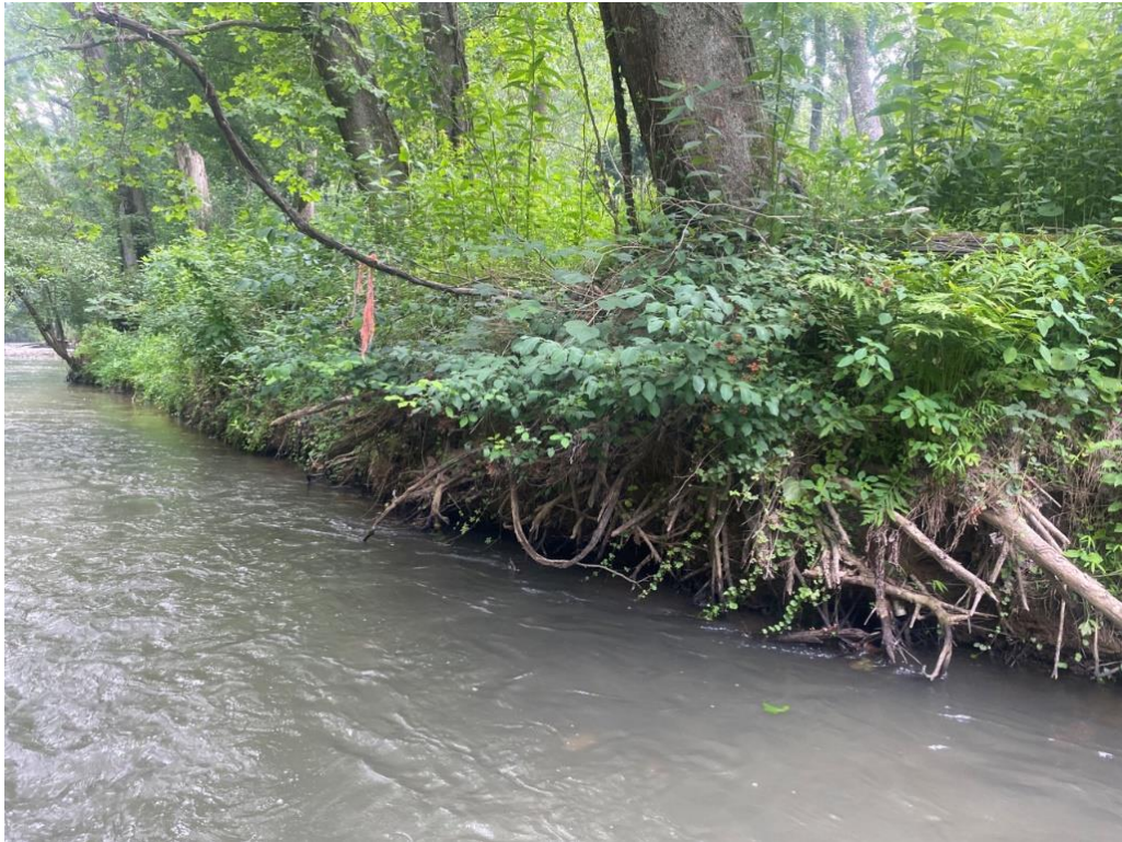
Erosion Area 3; Category “Moderate”
