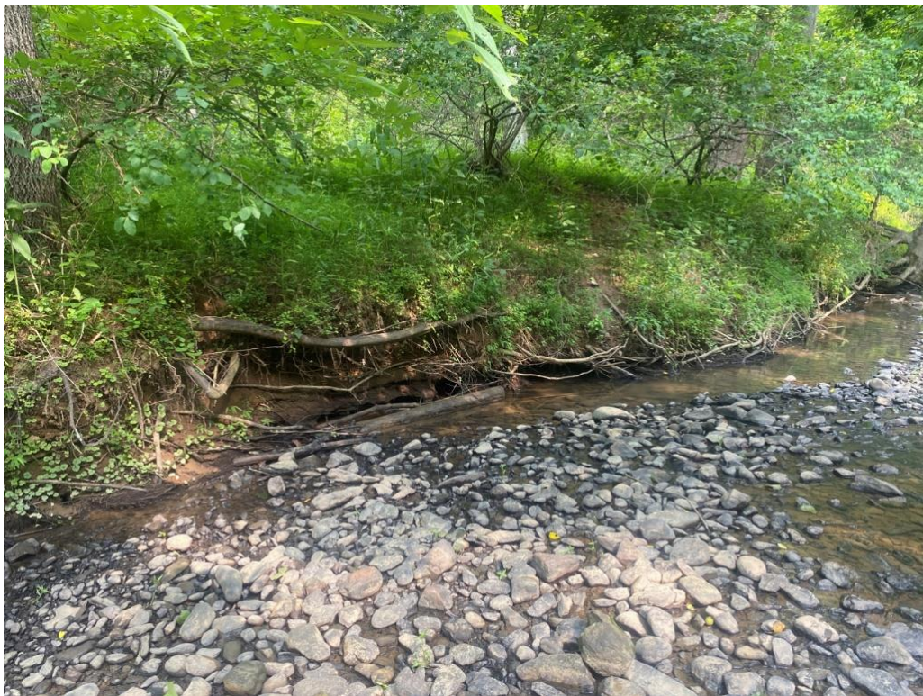
Erosion Area 2; Category “High”
