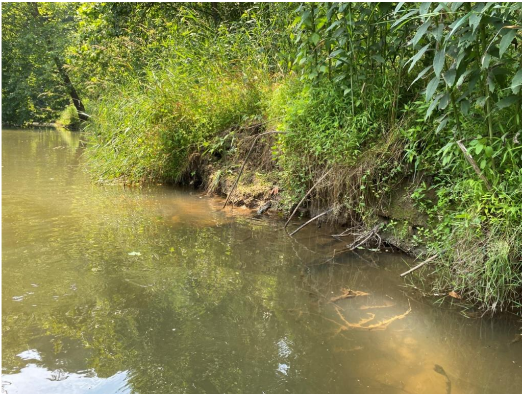
Erosion Area 14; Category “Moderate”
