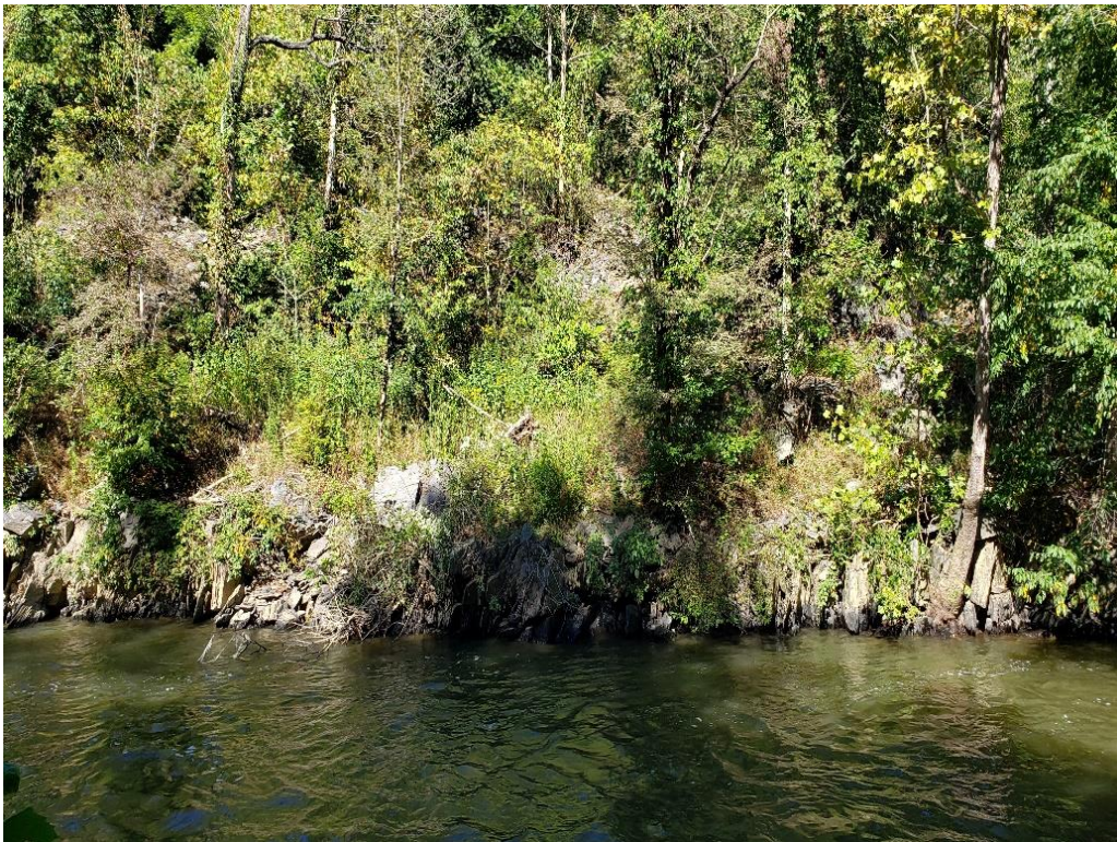
Erosion Area 8; Category “Moderate”
